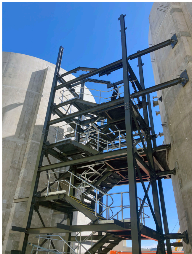
New access staircase being built between the digesters
