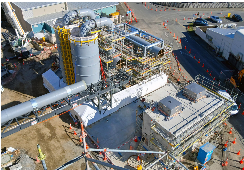
Above: The odour control system, pipe bridge and new ducting being installed.
